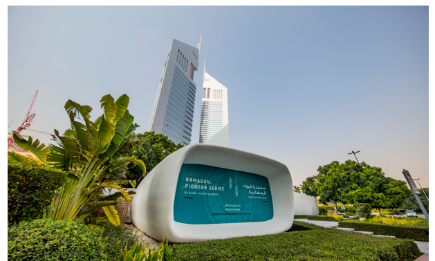
The Office of the Future was created out of concrete using a huge 3D printer
